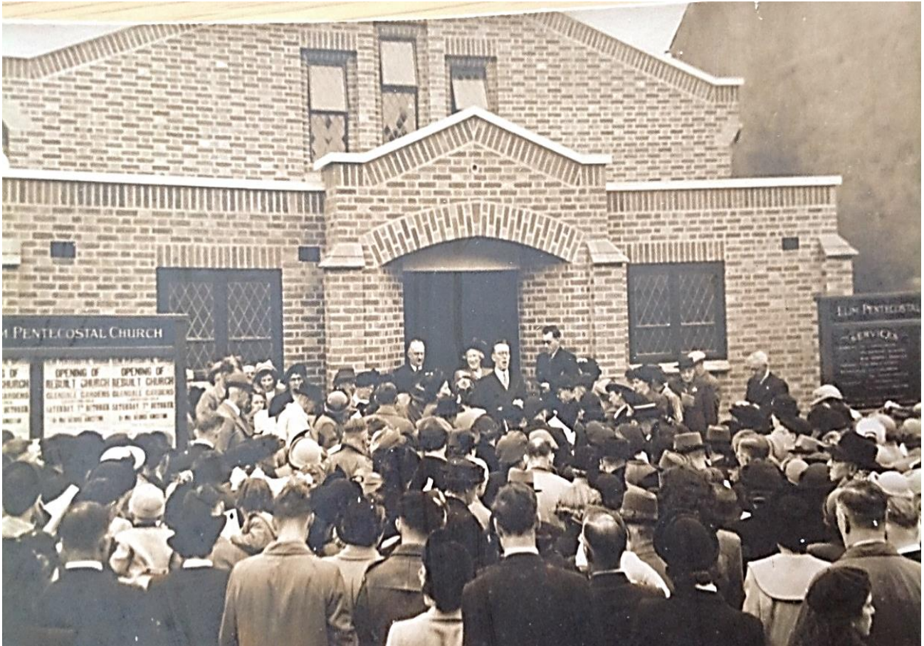
The opening of the new building
